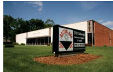
BOLTON & HAY 2701 DELAWARE AVE
